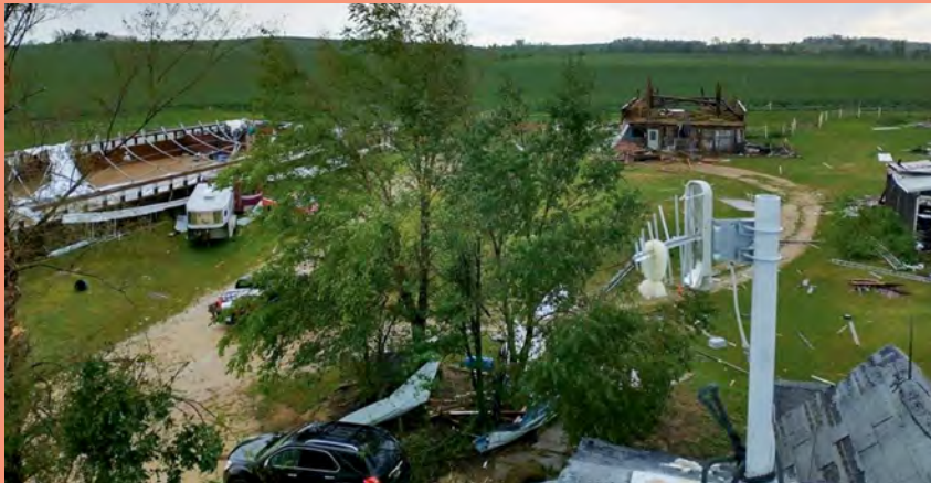
DEVASTATED: What was left of Tamarack Stables in Iowa after an August 2020 derecho
