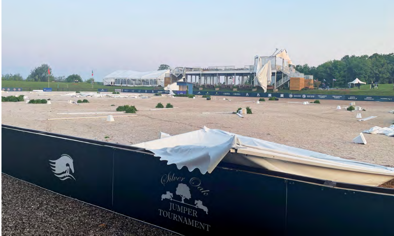
SET SAIL: Winds tore the tent material off the two-story VIP structure at the 2021 NAYC
